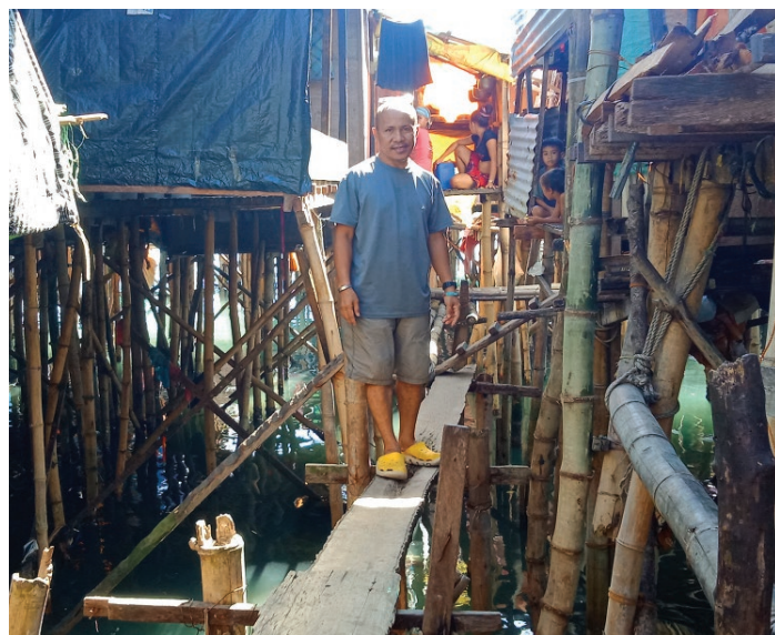
Pastor Bong leads the way across the shaky, single-board walkway.
