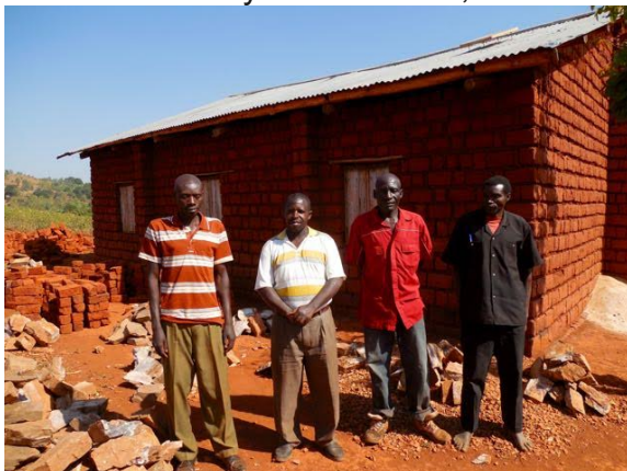
The remaining 4 elders at Munyinya church. The old church building is in the background and you can see the bricks and rock that have been gathered by the Christians for the new church building.
